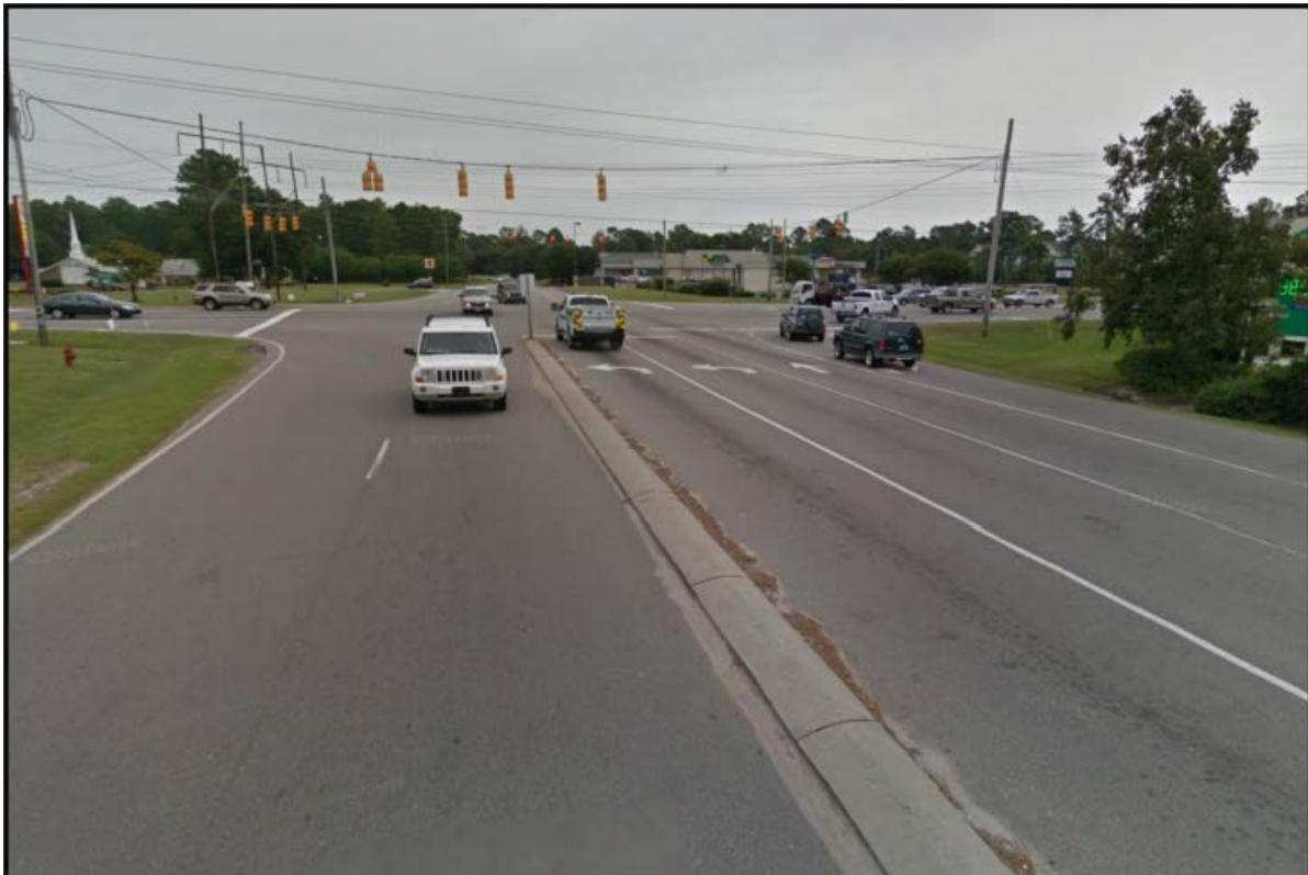
Google Maps (September 2012) – Looking East on SR 1322 (Bavarian Ln.) at US 117 - NC 132 (N. College Rd.)
