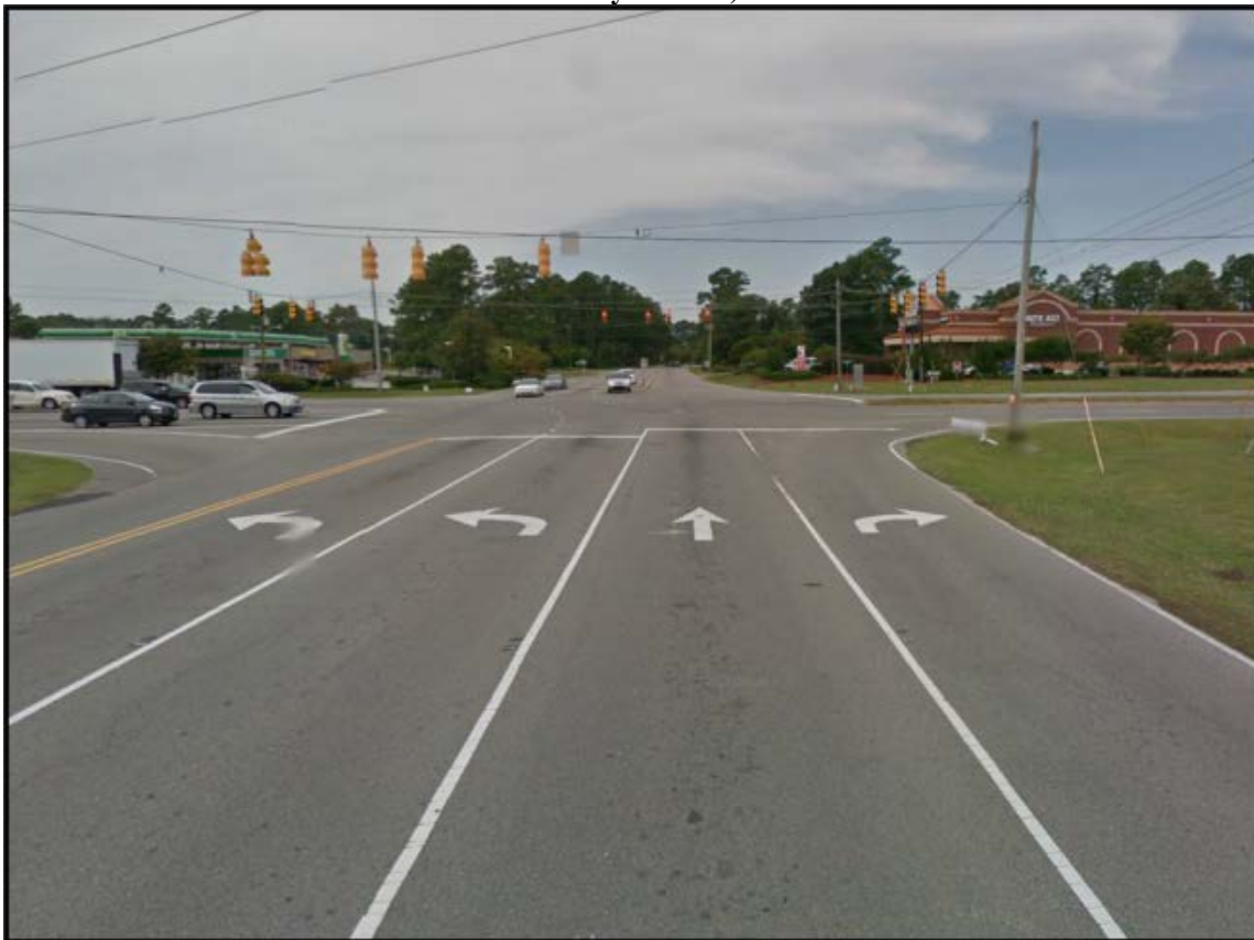
Google Maps (September 2012) – Looking West on SR 1322 (Murrayville Rd.) at US 117 - NC 132 (N. College Rd.)
