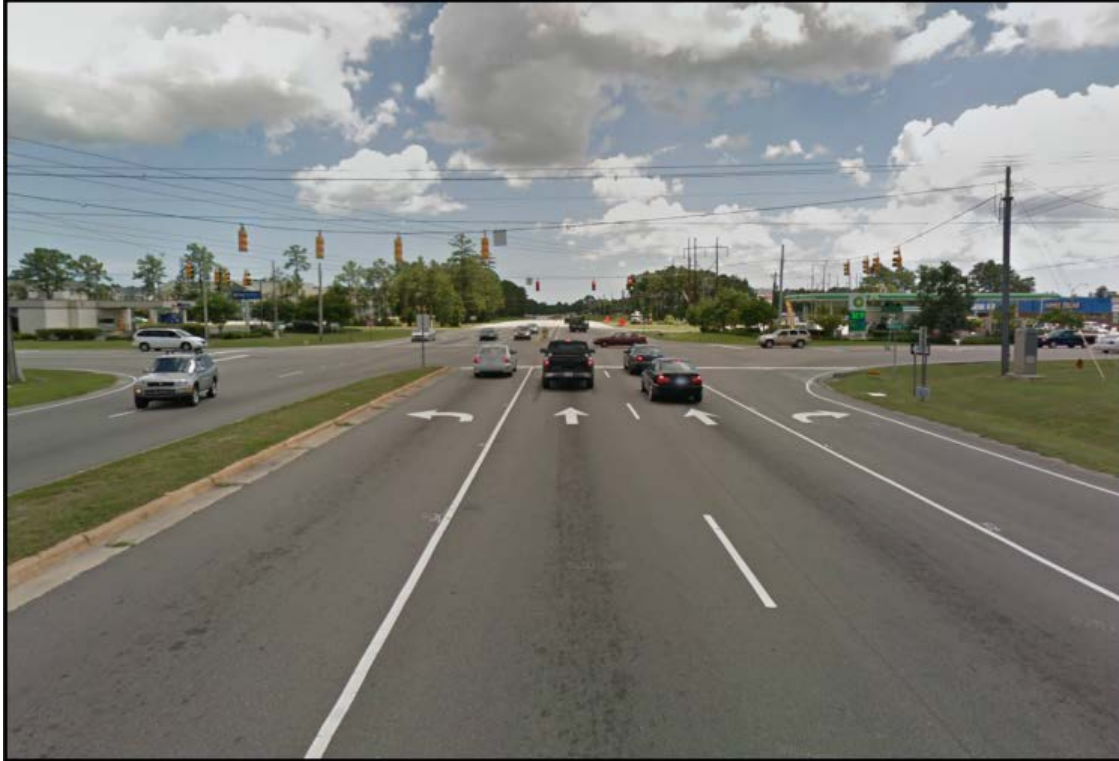
Google Maps (July 2012) – Looking South on US 117 - NC 132 (N. College Rd.) at SR 1322 (Bavarian Ln. / Murrayville Rd.)
